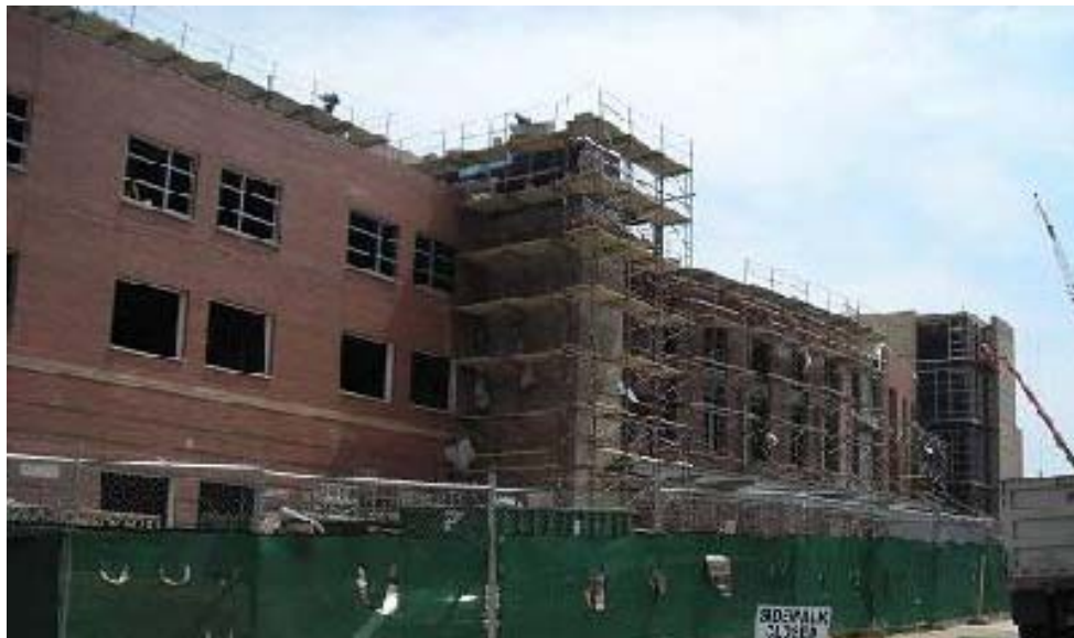
Scaffolding around the exterior of the school
